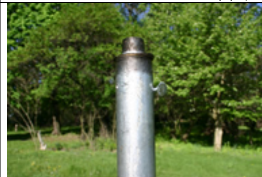
Narrow pipe should protrude a few inches
