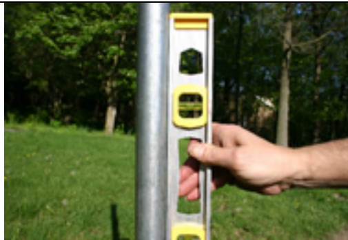
Make sure pipe is plumb
